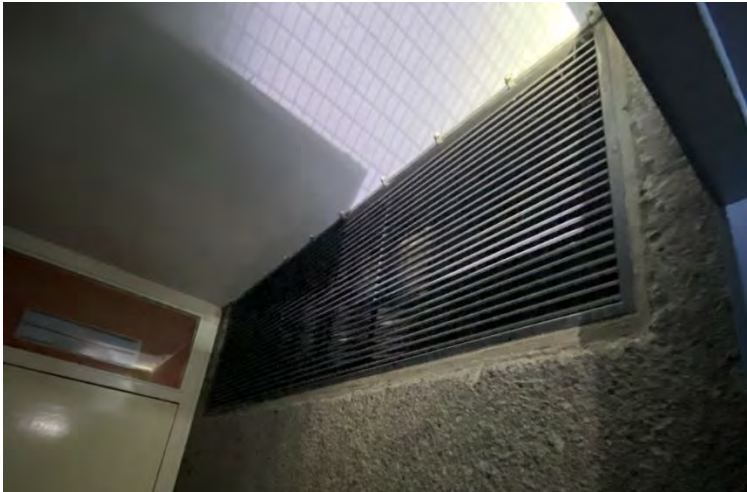
Figure 12: Louvre connecting the small lobby and the electrical riser The current arrangement of small lobby, firefighting stair, ventilation shaft and electrical riser is as shown in Figure 13.
